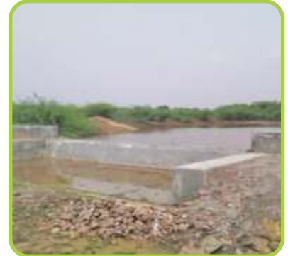
Pond renovation- Ruva
