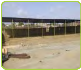
Hall renovation, Gajod
