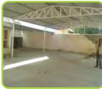
Hall renovation, Beraja
