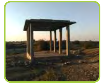
Crematorium renovation, Vadjar
