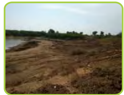
Pond renovation, Akwada
